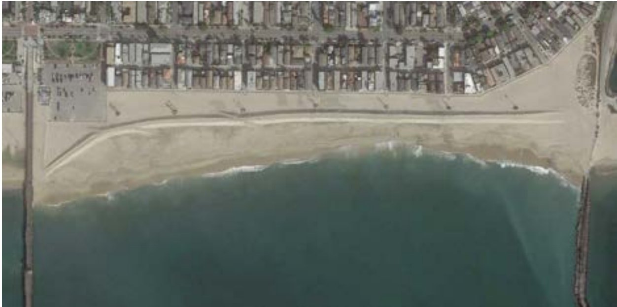
Figure 2-5: Satellite image of sand dike construction in winter 2017. (Photo credit Google Earth)
