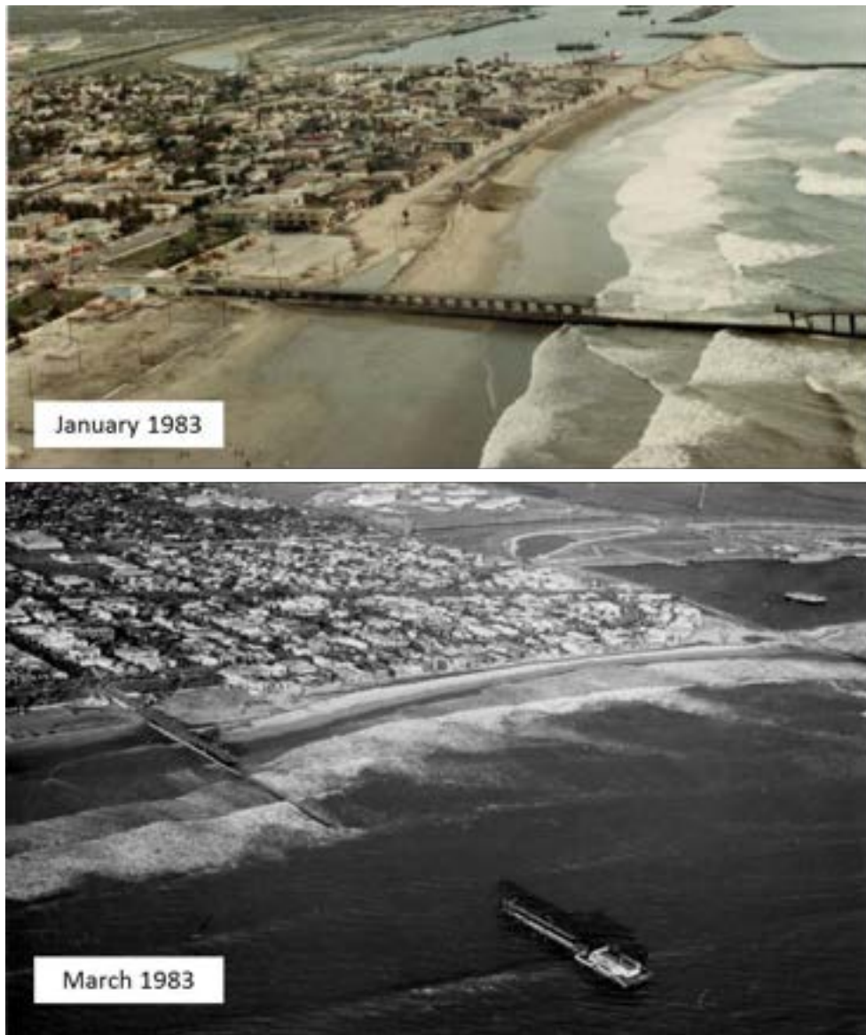
Figure 5-1: Damage to Seal Beach Municipal Pier during the winter of 1983.
