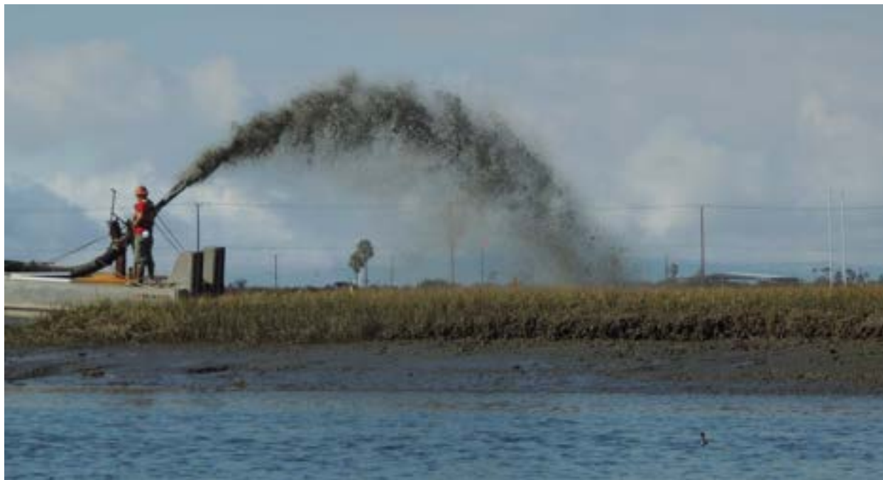
Figure 8-13: Thin-layer sediment placement within the Seal Beach National Wildlife Refuge (M&N, 2016)
