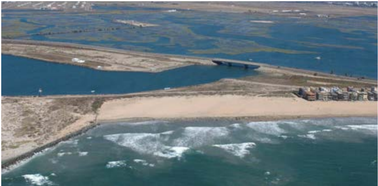
Figure 1-4: Eastern Seal Beach coastline featuring the Anaheim Bay east jetty, Pacific Coast Highway, and western border of the Surfside community (Copyright © 2008. Kenneth and Gabriel Adelman, California Coastal Records Project).
