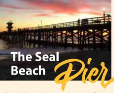
The Seal Beach pier was originally built in 1906, with a length of 1,865 feet, making it the second longest wooden pier in California. The timber pier consists of piles, longitudinal and lateral bracing, cap beams, stringers, blocking, decking and railing.
