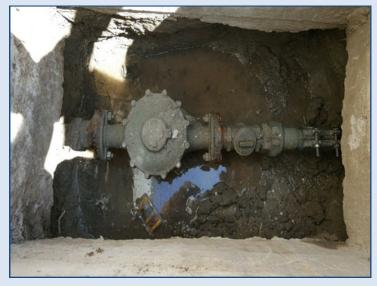
The City of Seal Beach Water Department has been on the hunt to find the shut off valve to a 2 inch water service on North Gate Road in Leisure World. The water operators had to do some potholing to find the valve in order to shut it off in case of a water line break. The valve was found which allows the water line to be isolated if need be. The next step is to patch the asphalt excavations and concrete.
