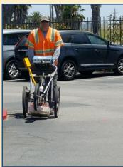
The City of Seal Beach Water Department has hired a construction company that has the capability to find underground utilities without excavating. The contractor will be using a ground penetrating radar to find underground utilities for a construction job taking in the place Eaves Apartments. The use of the
