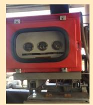
The city of Seal Beach Water Department installed new Murphy control panels to operate the electric and natural gas motors at the Bolsa Chica Well. The old
