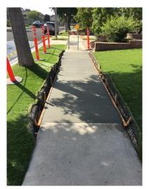
Working in between slurry seal projects, Public Works crews have been busy replacing sidewalks in need of repair. Sidewalks are removed and replaced over a short period, typically one to two days, to allow for pedestrian access over weekends. Nearby site conditions are always restored to pre-work conditions.
