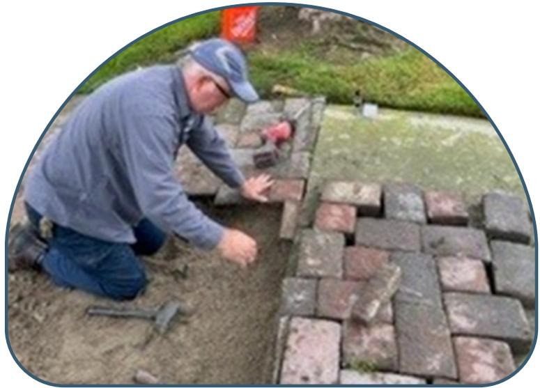
Staff repaired a cluster of pavers along the Electric Avenue greenbelt walkway that had developed an uneven surface. The pavers were removed and reset to ensure a level walking surface.
