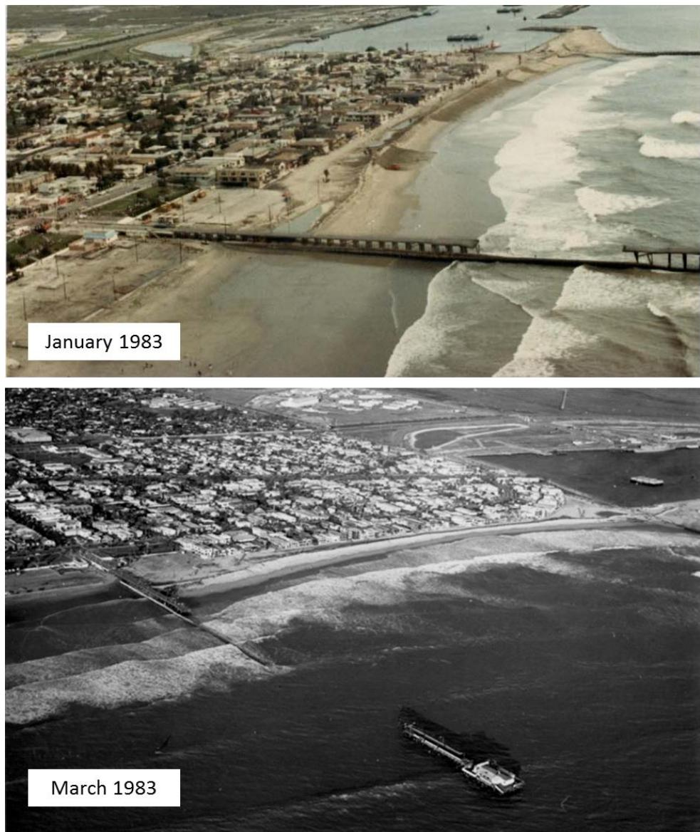
*Figure 5-1: Damage to Seal Beach Municipal Pier during the winter of 1983.*
