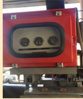
The city of Seal Beach Water Department installed new Murphy control panels to operate the electric and natural gas motors at the Bolsa Chica Well. The old
