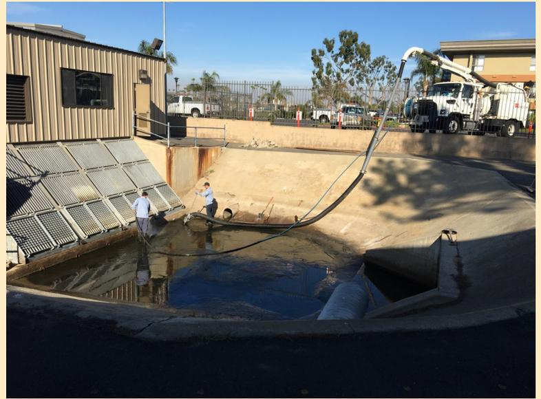
During last week's rain, the West End Pump Station's new trash rack was put to the test. This screen helped to protect the pumps by keeping debris from entering the pumping pit.
